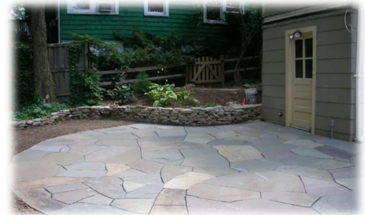
Irregular Bluestone Flagging Patio
