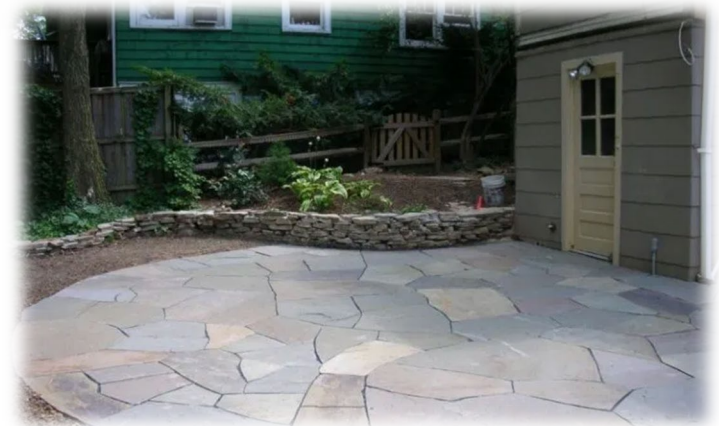
Irregular Bluestone Flagging Patio
